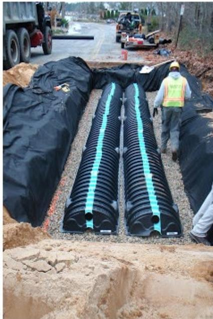
**FIGURE 13. Sub-surface Treatment Chambers**
