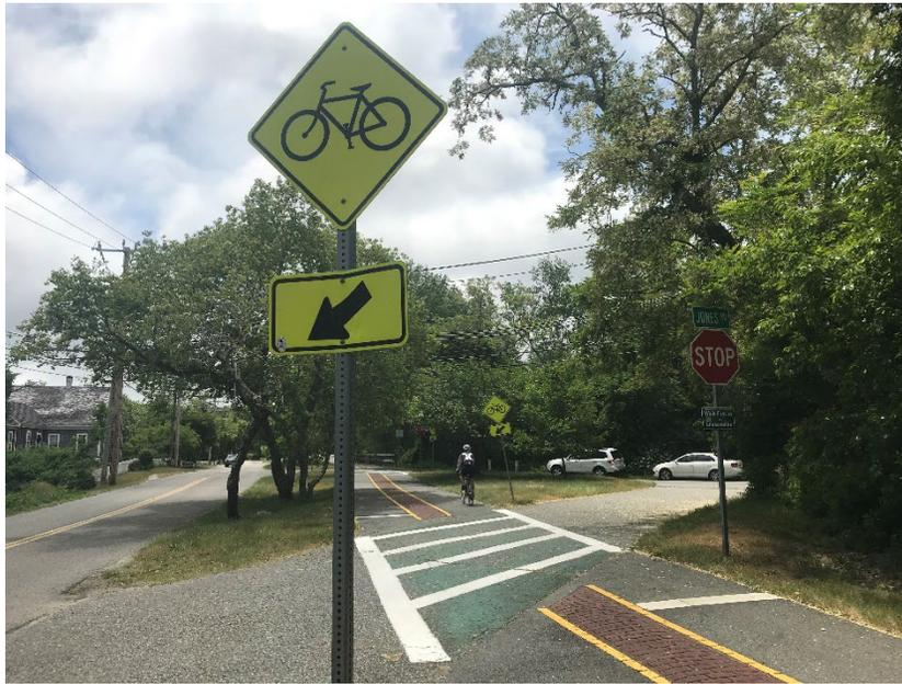
*Figure 102: Image of Path Crossing the Southern Leg of the Y Intersection (Jones Road). Note the Bike Trail Crossing Signage and Ladder Crosswalk*
