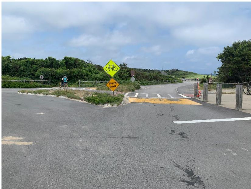
*Figure 86: Path Approach (Looking West). Note the Paint Delineating the Speed Bump*
