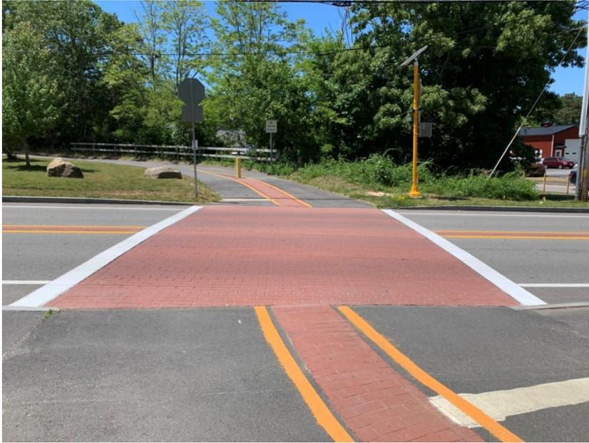
*Figure 122: Image of the RRFB, with Clear Pavement Markings*
