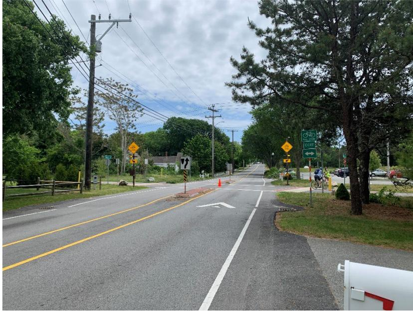
*Figure 199: East-Facing View of Path Crossing. Medians Provide a Place for Bicyclists and Pedestrians to Make 2-Stage Crossings*
