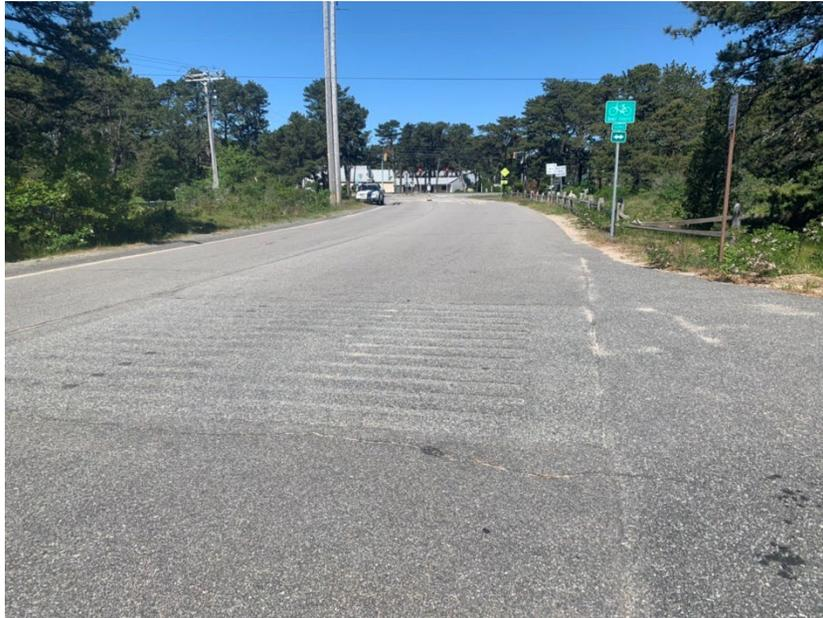
*Figure 66: Faded Paint is Used on the Crosswalk. Note the RRFBs.*
