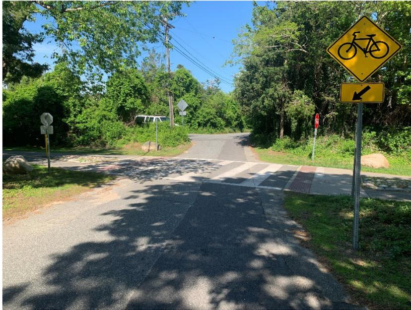
*Figure 43: Splitter & Post Decreases Chance of a Vehicle Turning onto Trail*
