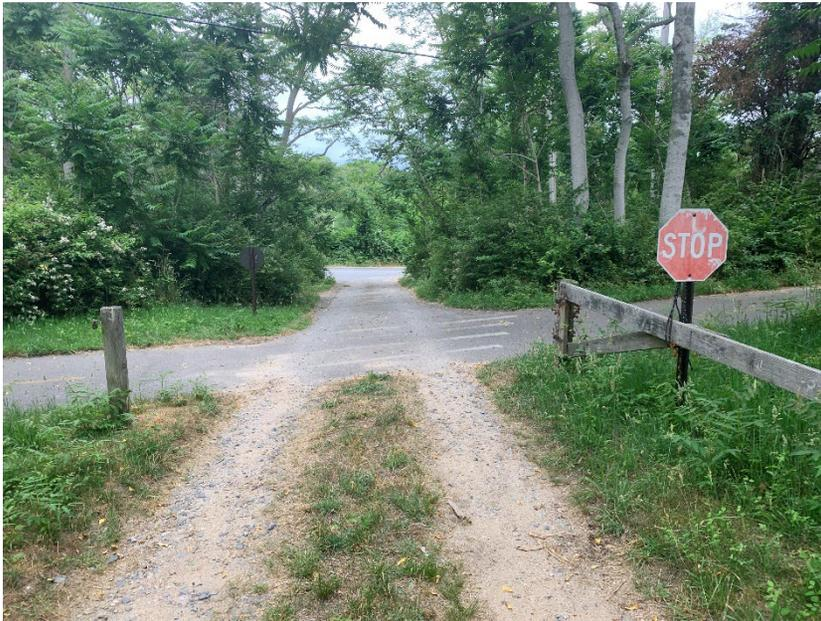
*Figure 94: Path Approach. Note the Faded Crosswalk Covered by Dirt from Passing Cars.*
