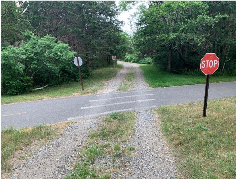
*Figure 92: Path Approach. Note the Faded Crosswalk Covered by Dirt from Passing Cars.*
