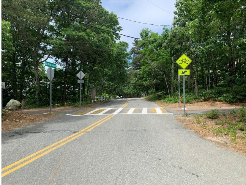
*Figure 130: Approach to Road Crossing with Splitter and STOP Control*
