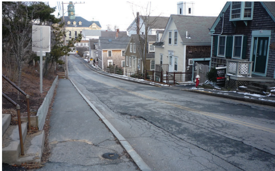
Buildings hug the road along Bradford Street near Prince Street in Provincetown
