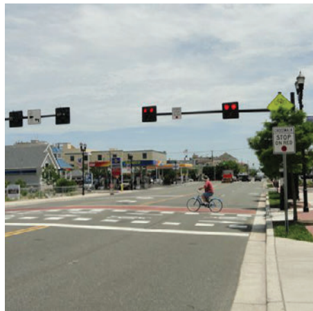
HAWK beacon http://ocnjdaily.com/ocean-city-activates-new-bike-crossing-signal/
