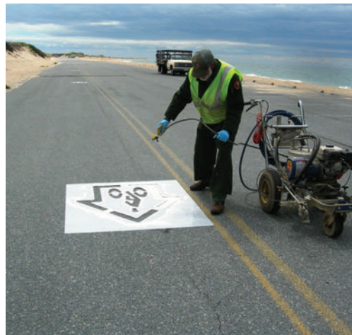
Adding a sharrow to roadway
