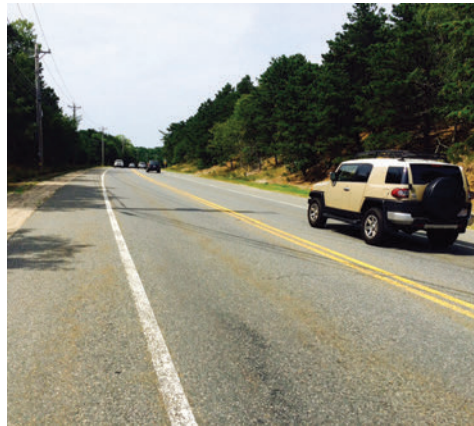
Paved shoulders on Route 6 in South Truro
