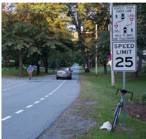
Advisory Bicycle Lane in Hanover, NH. Photo by Danny Kim, from The Dartmouth , September 25, 2014
