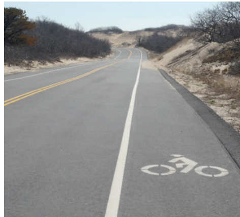
Bicycle Lane on Moors Road/Province Lands Road in Provincetown
