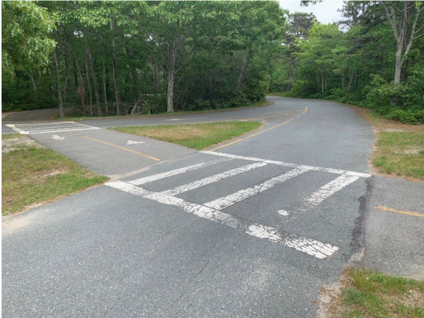
Figure 59: Road Approach (Note the 2-Stage Crossing).
