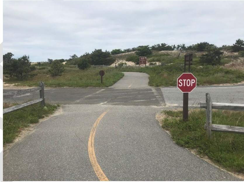
Figure 52: Path Approach to Crossing (Facing North)
