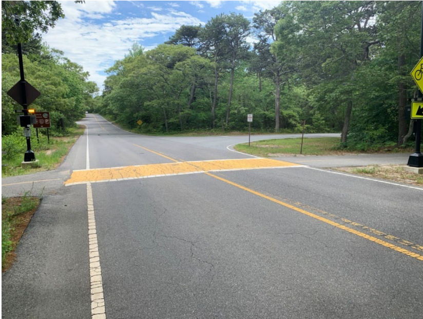
Figure 57: Road Approach (Note the RRFBs) and Painted Crosswalk
