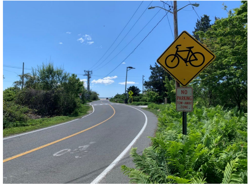
Figure 24: Advance Warning Signage with Faded Pavement Markings
