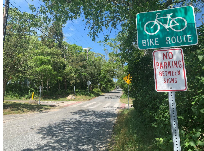
Figure 47: No Regulatory Signage in Advance of the Crossing
