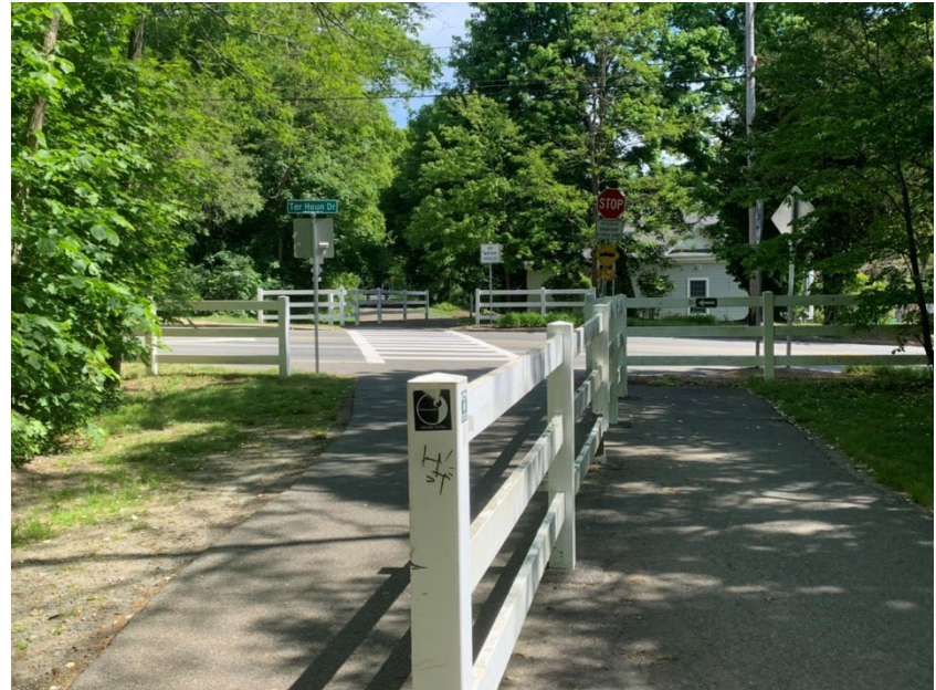
Figure 33: Bike Trail Approach at Ter Heun Drive (with Separator that Slows Bicycle Traffic)
