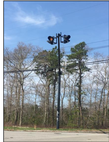
Image 1: Overhead flasher at Route 151 / Currier Road intersection
