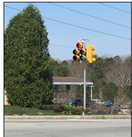
Image 8: Faulty traffic signal indications at the southwest corner of the intersection
