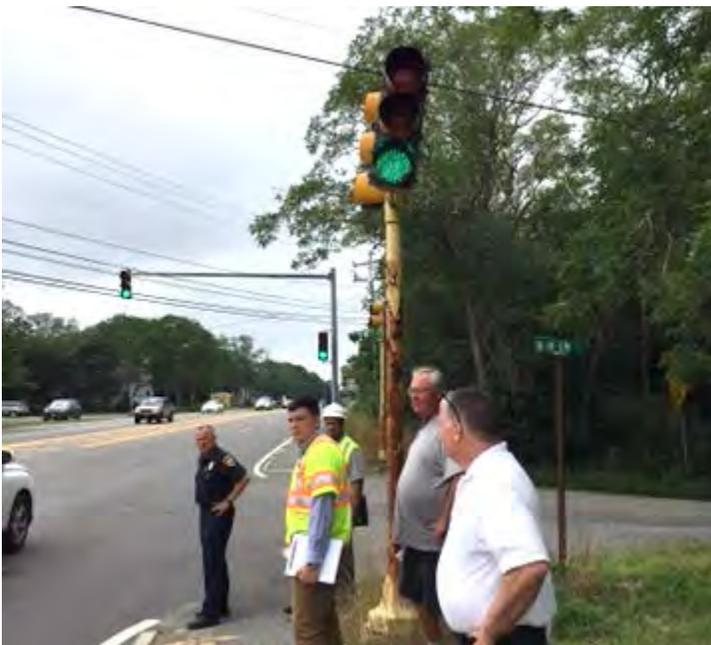
**Figure 7 - Route 6 southbound signal housing damaged and tilting**
