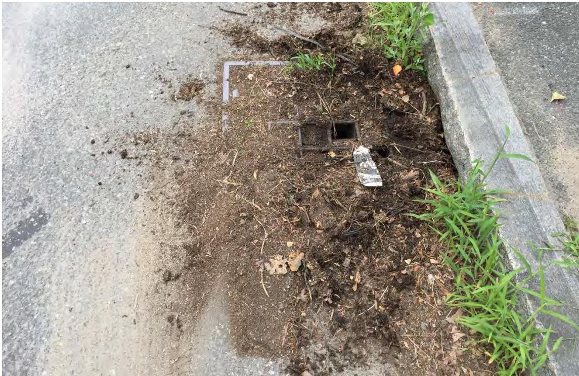
**Figure 15 - Catch basin blocked by debris**
