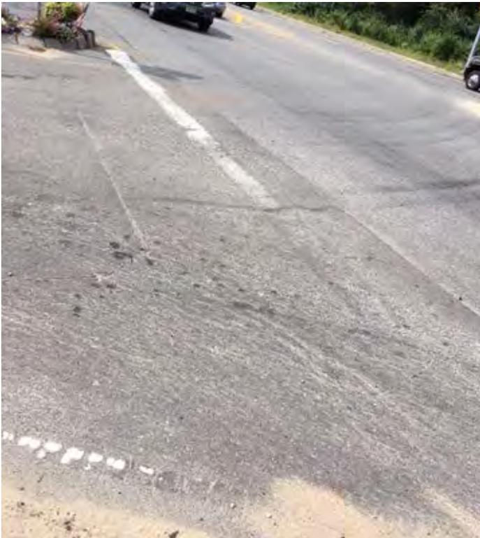
Figure 11 - Stop bar worn at Nauset Road approach
