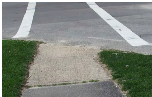
Existing Crosswalk Markings and Ramp
