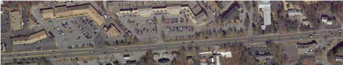
FIGURE 13 - AERIAL VIEW - ROUTE 28 CENTERVILLE FOUR-LANE SEGMENT - EXISTING CONDITIONS
