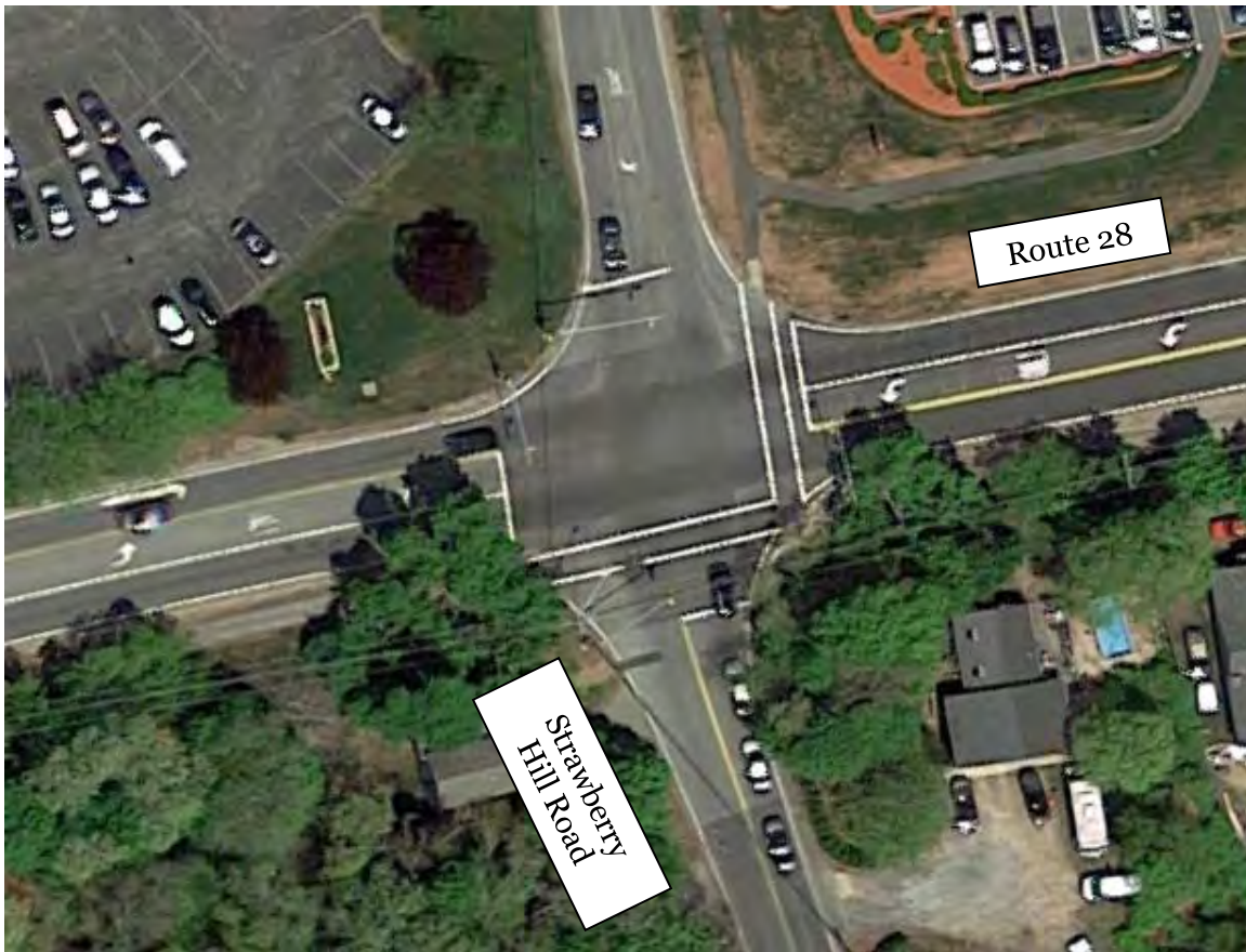
FIGURE 29 - ROUTE 28 AT STRAWBERRY HILL ROAD (AERIAL VIEW)
