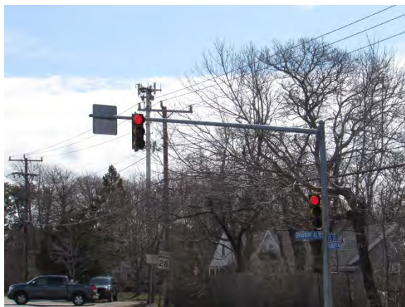
Lack of Backplates on Existing Signal Heads
