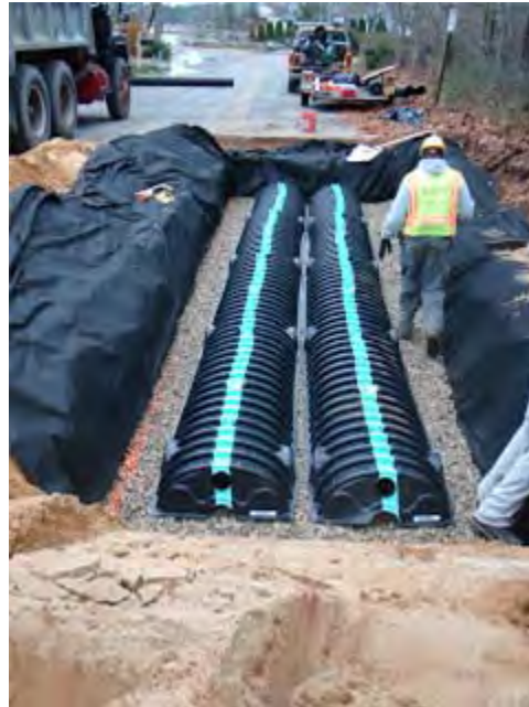
FIGURE 43 - HDPE SUB-SURFACE TREATMENT CHAMBERS
