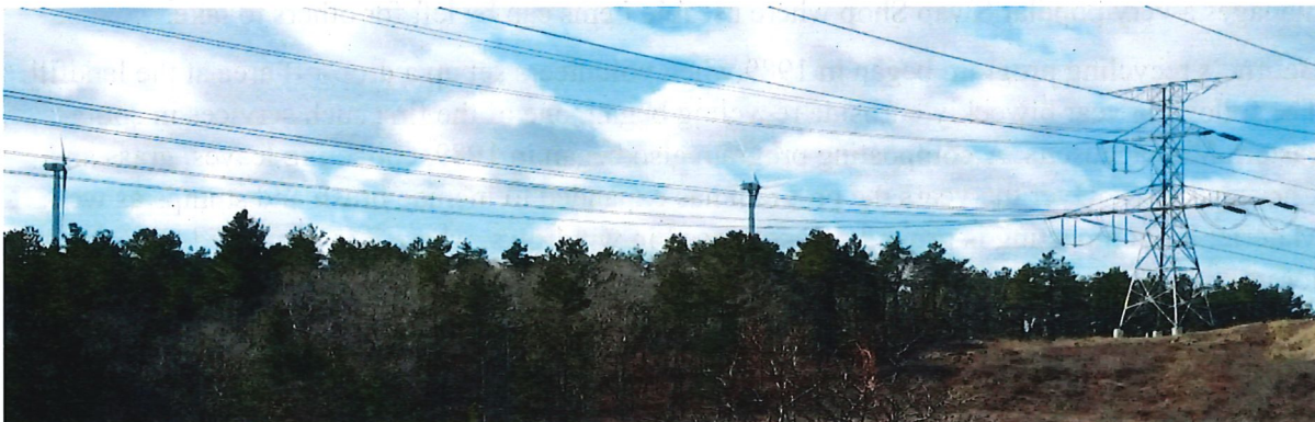
Sagamore Wind Turbines and Power Lines - Photograph by Wesley Ewell
