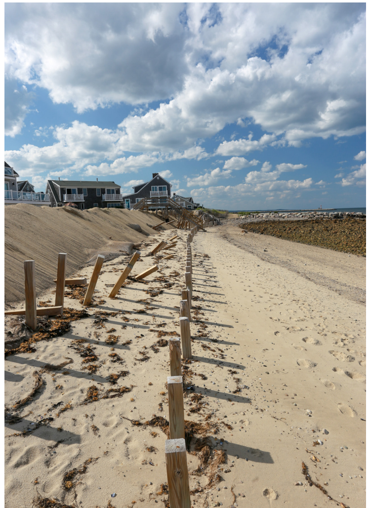
Coastal reinforcement at Town Neck Beach (photos left & right)
