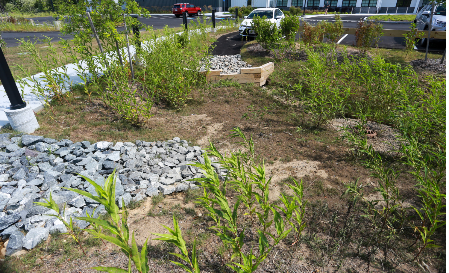
Stormwater retention basin at the Center for Active Living
