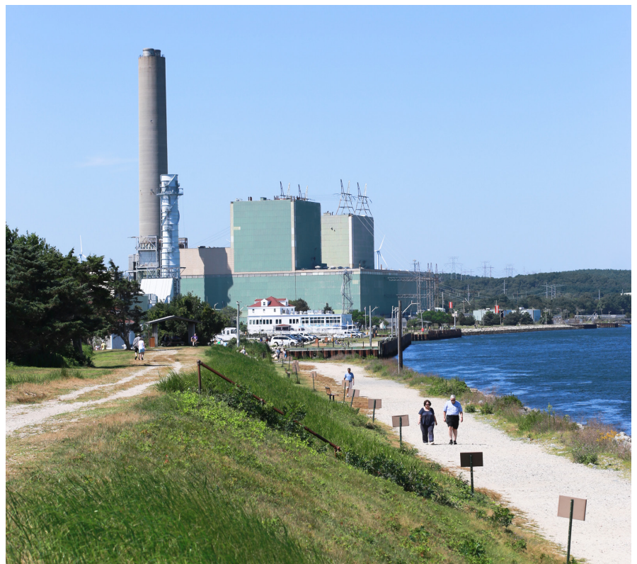
Canal Station Power Plant
