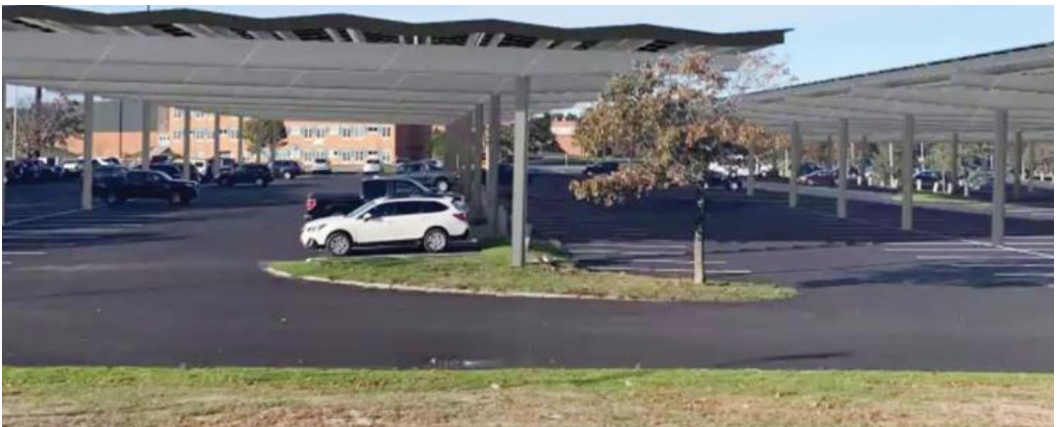
Proposed solar array at (top) Sandwich Hollows Golf Club and (bottom) Sandwich High School.
