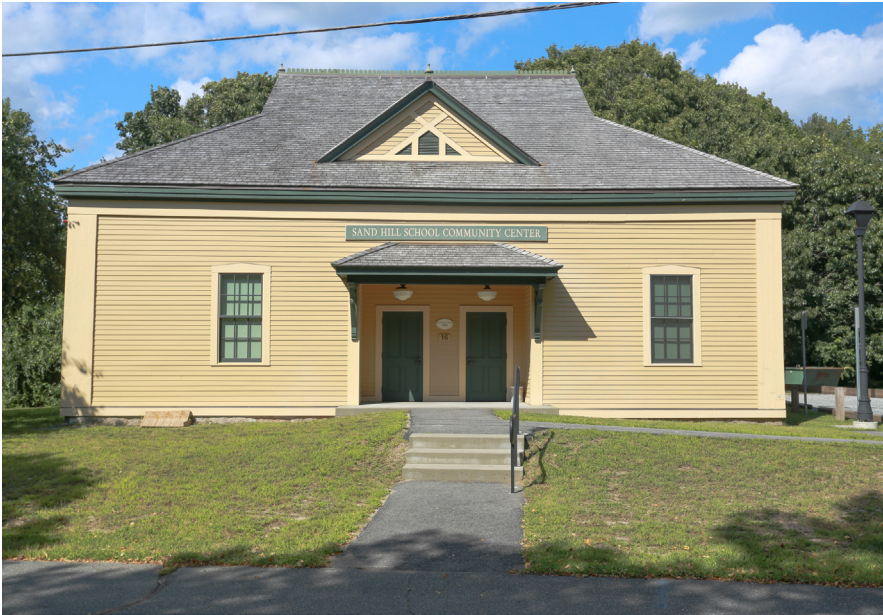
Restoration of the Sand Hill School Community Center (2018)
