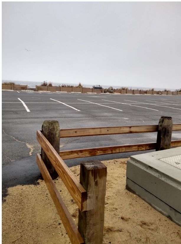
Photograph 2: Paved parking area, facing south
