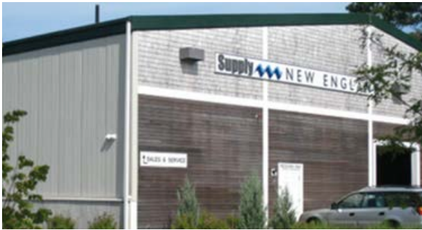
Figure 9 This building in Yarmouth uses a mix of traditional materials on the most visible facades and low-reflective siding in neutral tones on the side facade.
