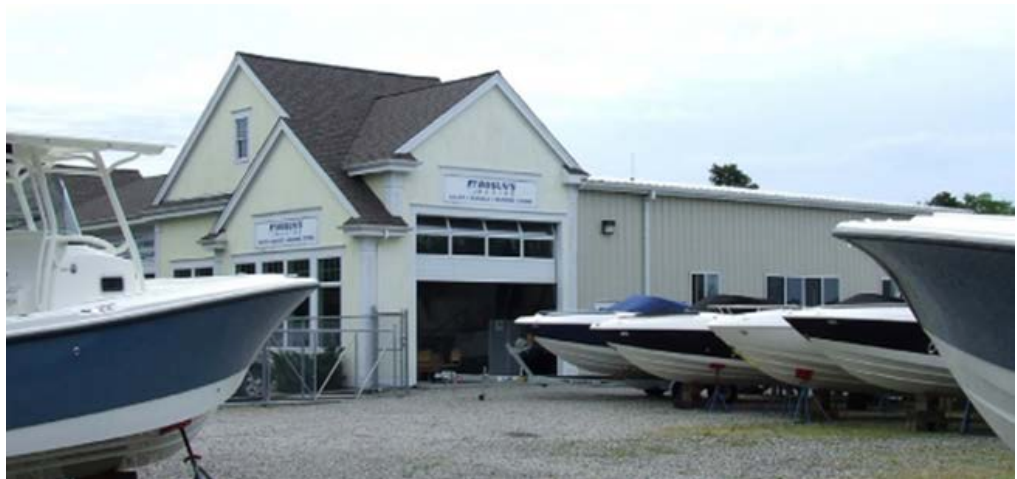
Figure 20 At this marine-supply retailer in Mashpee, a metal warehouse structure has been attached to the rear of a building with a more traditional form.
