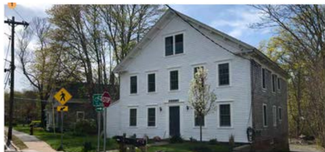
Figure 6-37. Sandwich manor house presents a strong face to the street and discreetly shields parking behind.
