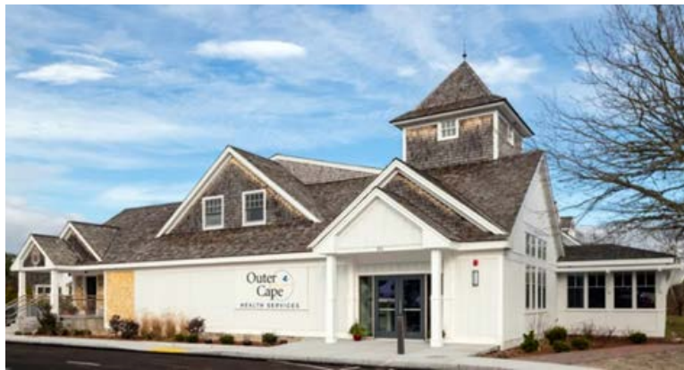
Figure 4 The Outer Cape Health Services facility in Harwich uses varied eave lines and ridge heights to reduce the apparent mass of the building. (Delphi Construction, 2023)
