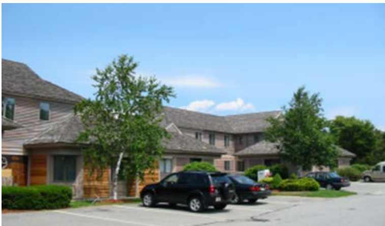
Figure 3 The varied wall heights on this traditional building reduces the visible bulk on a large structure. (Cape Cod Commission, 2009)
