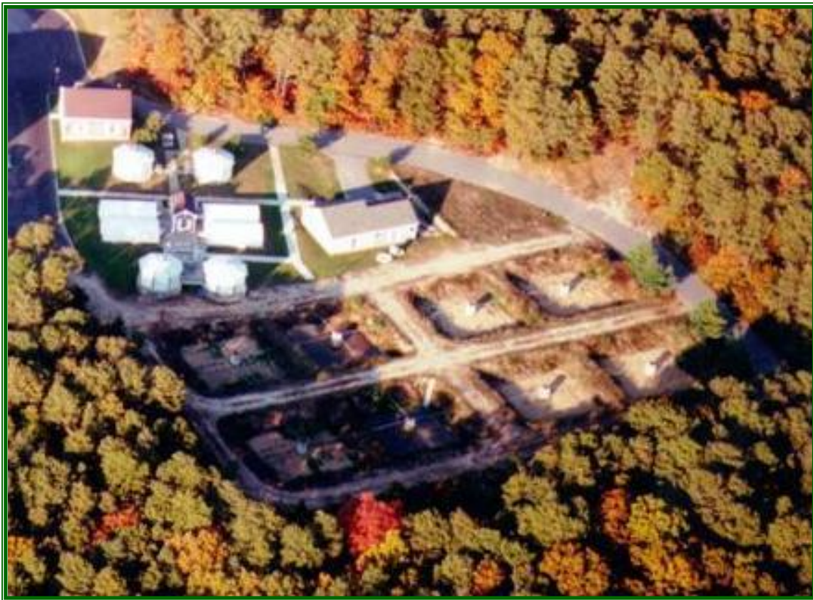
FIGURE 5-2 TRI-TOWN SEPTAGE TREATMENT FACILITY
