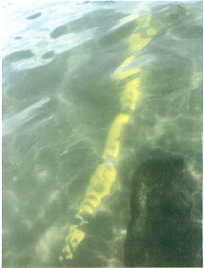
An exposed section of the transmission cable is seen here about three feet below the water at low tide. Courtesy photo
