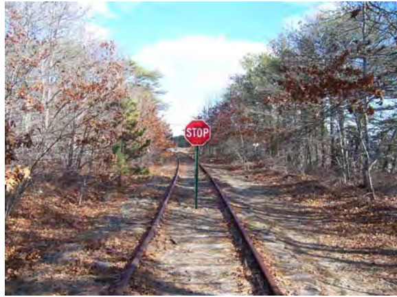
FIGURE 14: RAIL TRACKS IN YARMOUTH WEST OF STATION AVENUE. ALONG WITH THE STOP SIGN, STOPPERS ON THE TRACKS PREVENT TRAINS FROM GOING TOO FAR.
