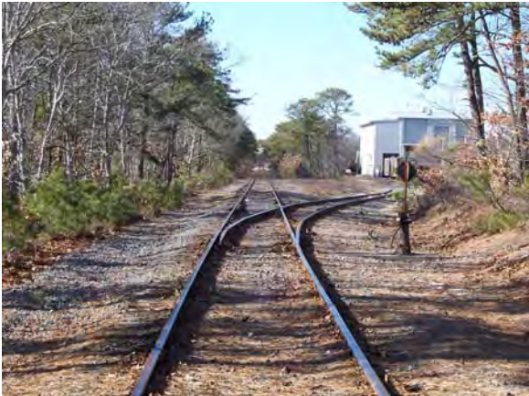
FIGURE 13: RAIL TRACKS IN YARMOUTH, FACING WEST. THE SHINY METAL SURFACE OF THE RAIL TRACKS INDICATES THEIR CONTINUED USE.
