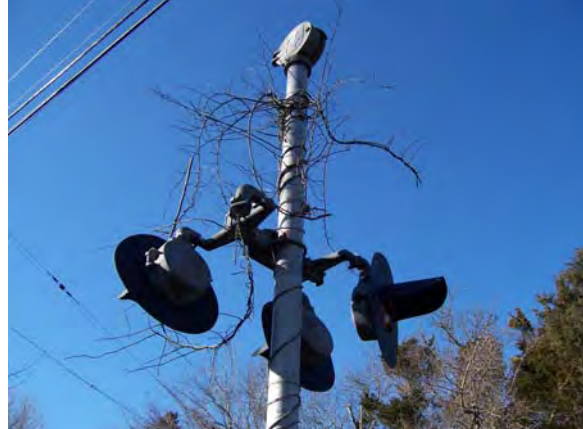
FIGURE 25: A CROSSING SIGNAL AT OLD DOCK ROAD OVERGROWN WITH VEGETATION
