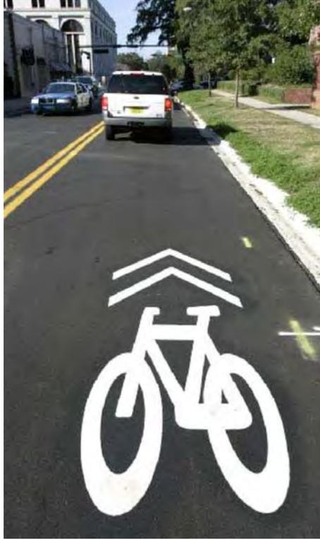
FIGURE 5 - "SHARROW" PAVEMENT MARKING
