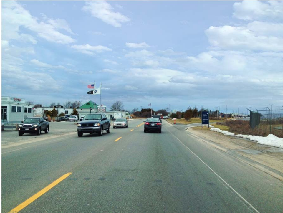
FIGURE 41 – BEFORE: ROUTE 28 EAST APPROACH TO AIRPORT ROTARY
