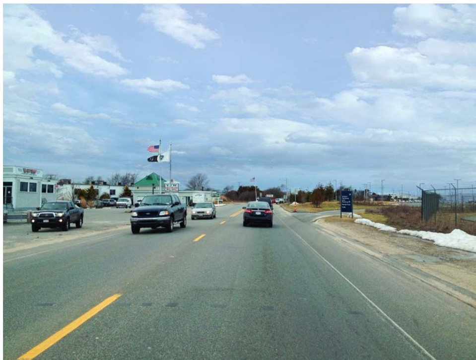
BEFORE: Route 28 East Approach to Airport Rotary
