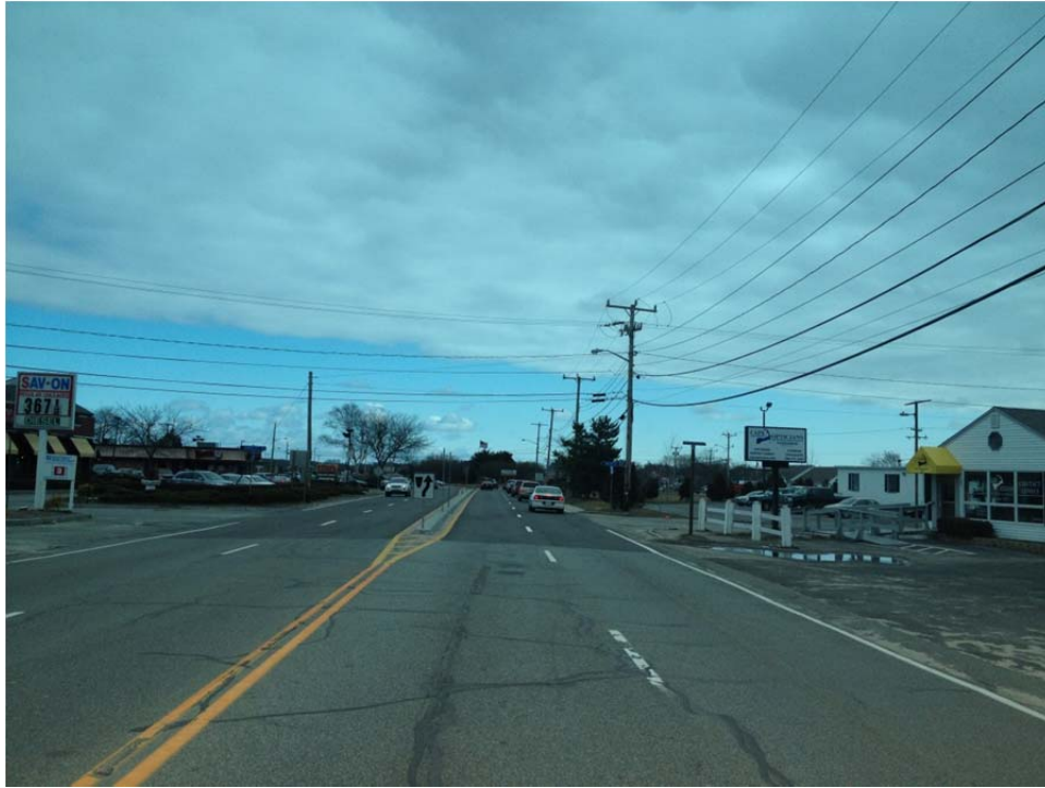
FIGURE 43 - BEFORE: ROUTE 132 APPROACH TO AIRPORT ROTARY
