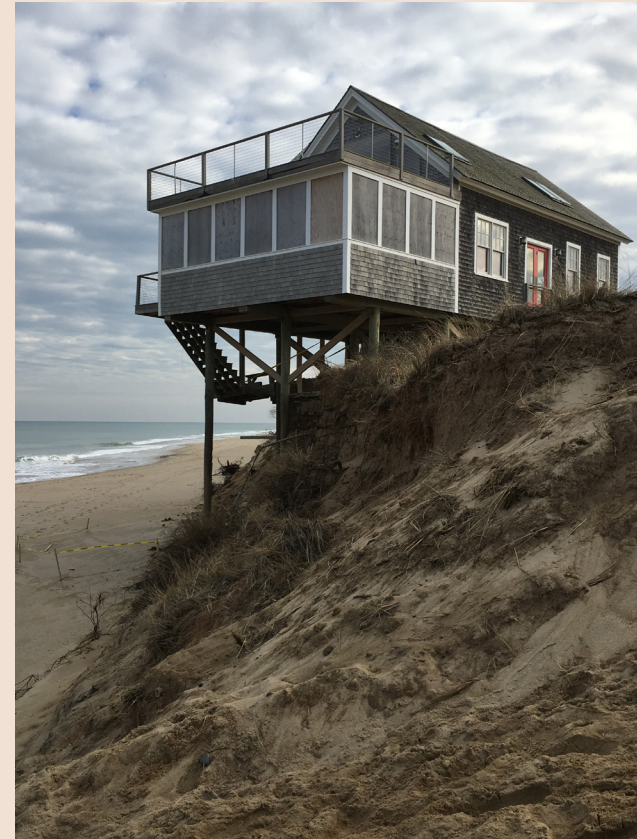
This Truro building and another next door were relocated farther inland to move them away from the eroding coastal bank and flood hazard areas.
