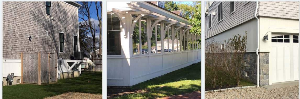
Building retrofits include elevating mechanical systems (left), filling basement areas, dry floodproofing (center), wet floodproofing (right), and elevating the interior first floor.
