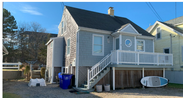
Small side addition to house mechanical equipment in an elevated interior space.
