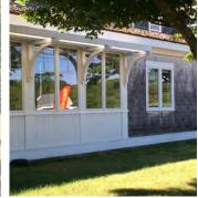
The lower portion of this building is a concrete water barrier covered with shingle siding and paneling to maintain the building's character.
