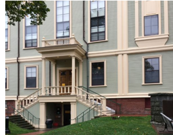
Provincetown Town Hall with lower entry stairs, doors, windows.
