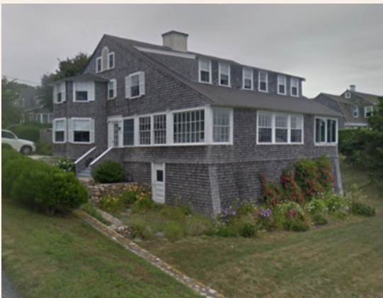
Historic Bourne and Hyannis Port buildings with inset shingle walls below base floor height, extended stairs, and landscaping.
