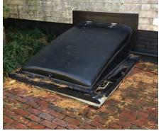
Tracks for drop-in flood barriers at ground-level doors (shown on left in building photo); water-tight exterior bulkhead over cellar access point.
