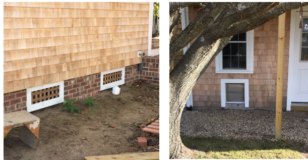
Flood vents allow water to flow in and out of unfinished and finished living spaces.
