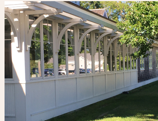
The original part of this historic house in Sandwich was wet floodproofed while additions were elevated to address flood risk (top); dry floodproofed office building in Harwich (bottom).
