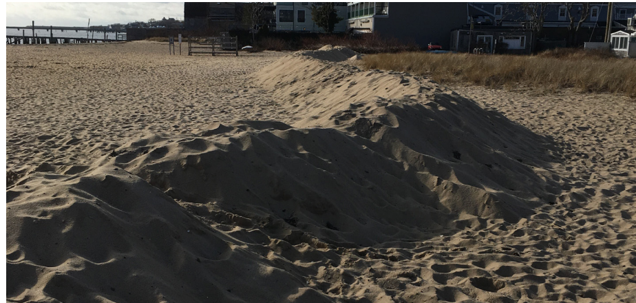
A temporary dune barrier blocks a storm tide pathway and protects the area around Gosnold Street in Provincetown.
