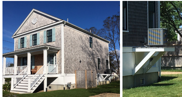
Raised platform on rear portion of side elevation for elevated mechanical equipment.
