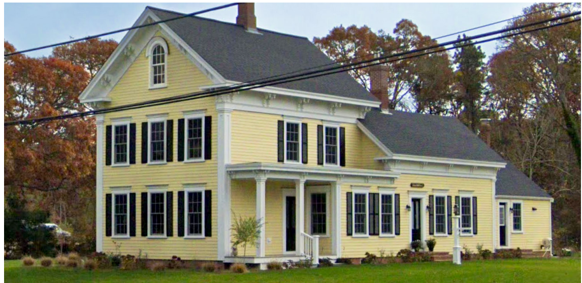
This historic building in Harwich was elevated several feet while preserving all its historic architectural features and trim details. Landscape materials were used to disguise the increased foundation height.
