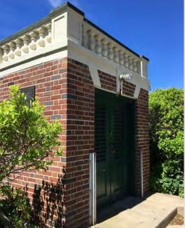
Historic structure on left with masonry walls below flood level. Entry could be protected with drop-in flood shields without changing entry style or detailing, as with building on right.
