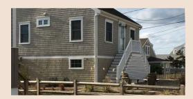
This elevated building includes architectural trim at the original base of the siding to illustrate the building's original scale. Different materials below the architectural trim would highlight the change even further. The enclosed basement area includes corner boards and window forms that complement the building's original details.
