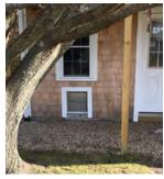
Flood vents allow water to flow in and out of unfinished and finished living spaces.
