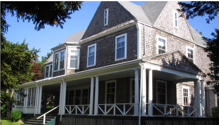
This Falmouth home was relocated from Chappaquoyt Island to North Falmouth to save it from demolition
