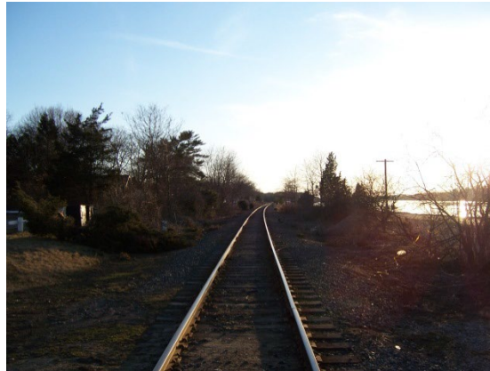
FIGURE 29. Rail Tracks West of the Sagamore Bridge
