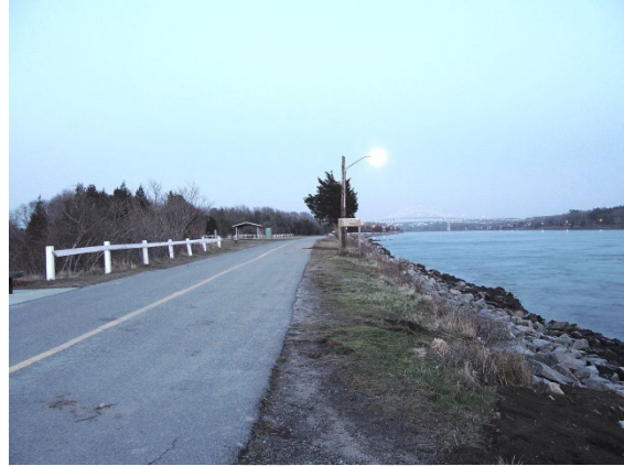
FIGURE 10. Mainland-Side of the Canal Bicycle Path, East of Railroad Bridge
