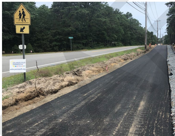
FIGURE 18. Phase 1 construction of the Higgins Crowell Shared Use Path
