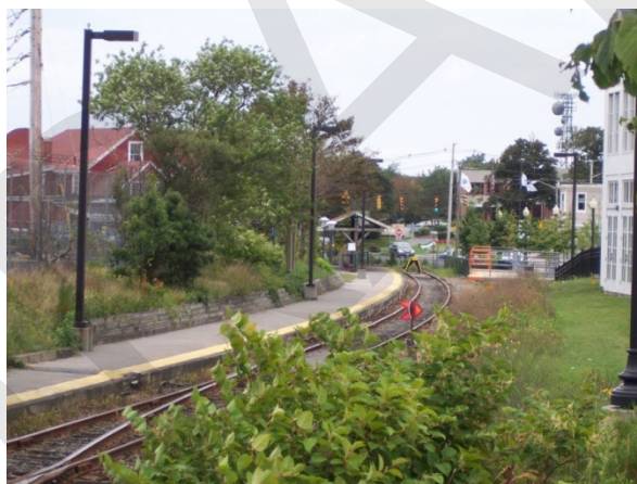
FIGURE 31. Rail Platform at the Hyannis Transportation Center
