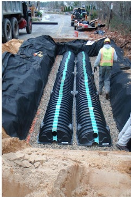
FIGURE 13. Sub-surface Treatment Chambers (Source: Lindsay Cook, Cape Cod Conservation District Intern)
