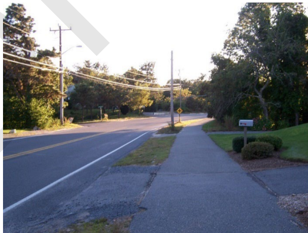
FIGURE 14. Setucket Road Path East of North Dennis Road, Looking West
