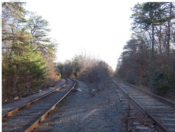
FIGURE 33. Rail Tracks at the Otis Junction
