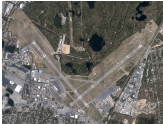
FIGURE 35. Barnstable Municipal Airport
