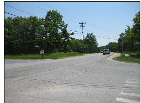
Grading changes between Great Neck Road North and Old Barnstable Road.
