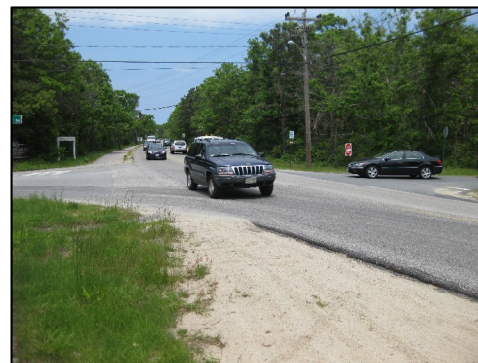
Worn pavement markings at the Great Neck Road North/Old Barnstable Road intersection.
