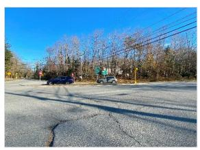
Image 9: Route 6A at Route 132 intersection; there are no inner shoulder or lane pavement markings.
