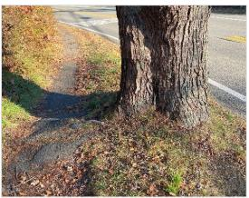
Image 7: Overgrown tree roots penetrating the sidewalk along Route 6A.
