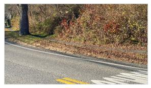
Image 12: Existing condition of sidewalks along the opposite side of Barnstable Elementary School on Route 6A. Sidewalks are extremely narrow, uneven, and close to the roadway.
