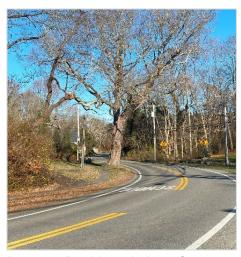
Image 3: Dashboard view of horizontal road curvature on Main Street (Route 6A) at Aunt Hatch Lane. In this location, vehicles often have trouble maneuvering the turn and cannot fully see roadway behind the curve.
