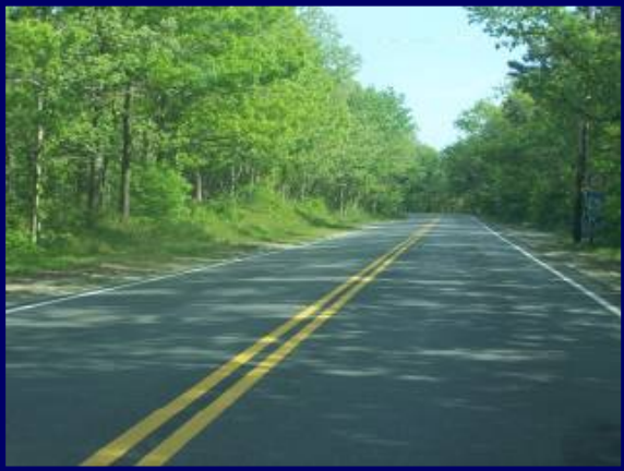
Figure 2. View of Route 130
