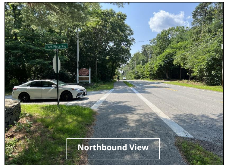
Signage South of Crossing
