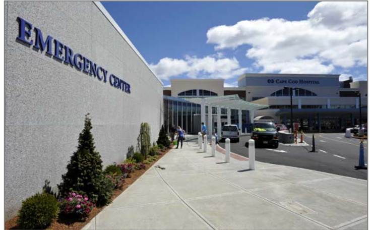
Figure 22. Recently Expanded Cape Cod Hospital Emergency Center
