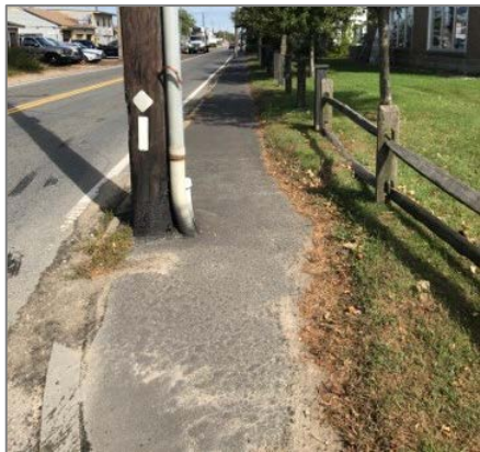
Figure 5. Existing Condition of Pedestrian Facility
