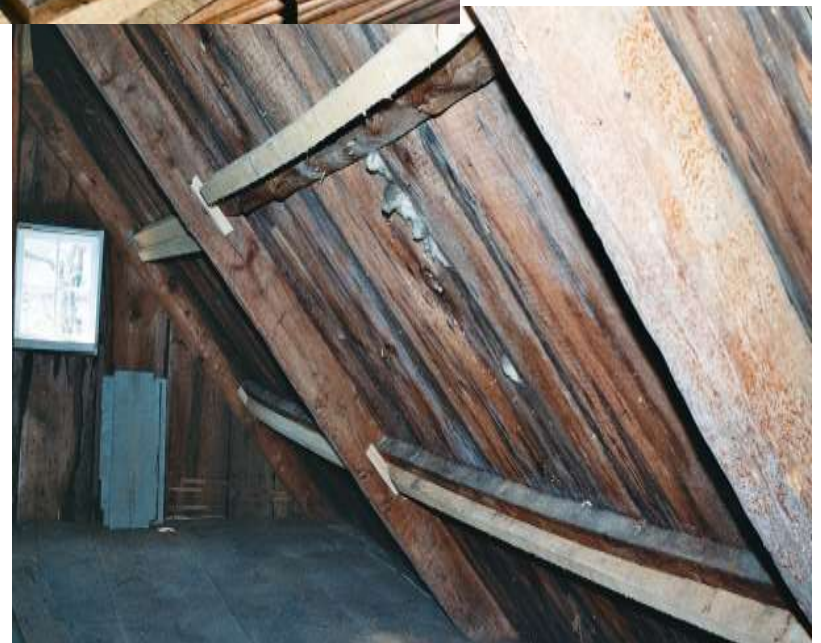
TYPICAL UNDERSIZED PURLINS Sistered with white oak and blocks
