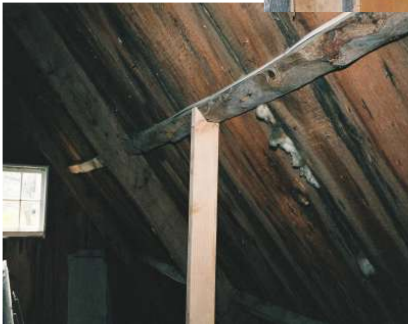
TYPICAL UNDERSIZED PURLINS Sistered with white oak and blocks
