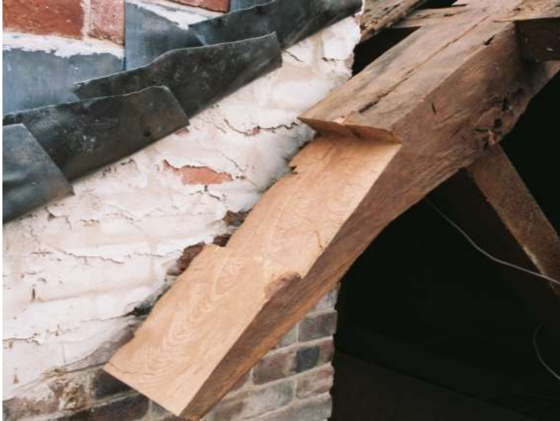
Existing Rafter Repair
