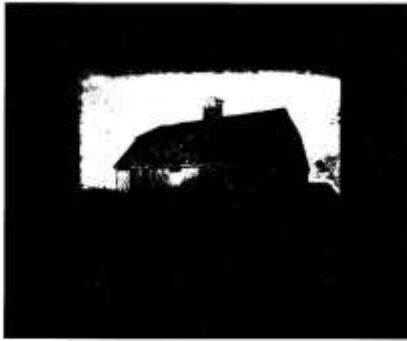
Atwood House Roof Structural Survey Chatham Historical Society 347 Stage Harbor Road Chatham, Massachusetts
