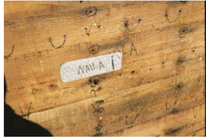
Extensively nailed mustard clapboards
