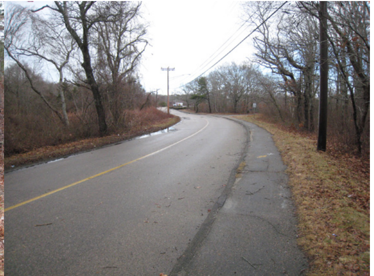
Spring Bars Road approaching the site, looking east.
