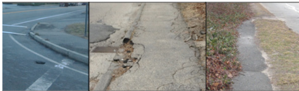
EXISTING ASPHALT SIDEWALKS
