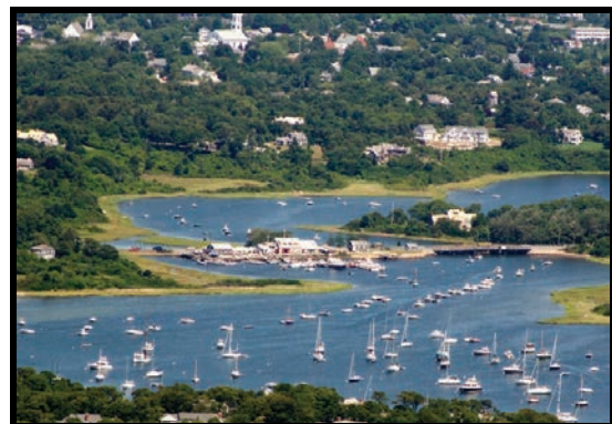
View of the Mitchell River, Stage Harbor Marine, and the Mitchell River Drawbridge (Photo by Amie Schaeffer)
