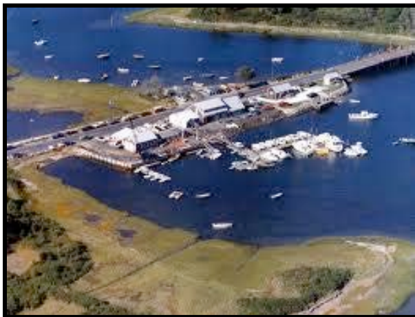
View of the Mitchell River Bridge and Chatham Marine (Courtesy of Town of Chatham)
