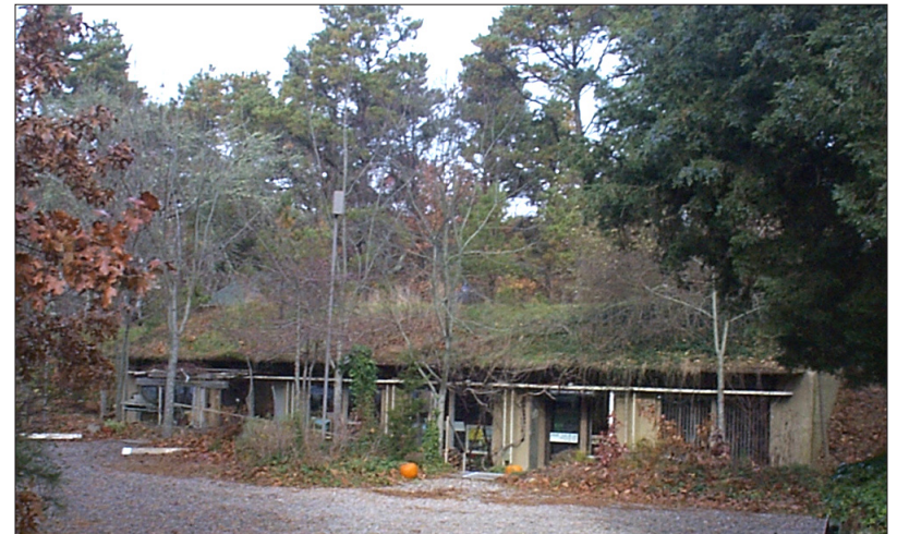
Figure B38: This residential home and studio in Brewster incorporates a “green” or “living” roof that supports soil and plant material that insulate the building and reduce heat absorption.
