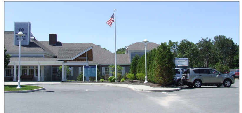
Figure A43: At a medical center in Harwich, the delivery area (right) is shielded from the public entrance to the building (left) by a narrow, but dense screen of trees (center right).
