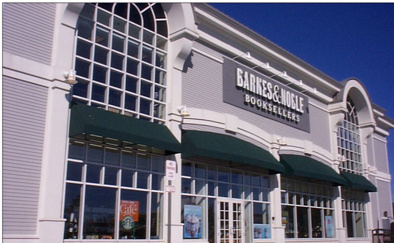
Figure B30: Windows and awnings oriented to pedestrians lend a human scale to larger buildings at the Cape Cod Mall in Hyannis.
