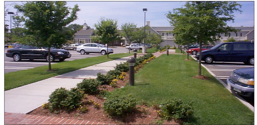
Figure A38: Wide landscaped islands with sidewalks provide a visual break, a pedestrian refuge, and an opportunity to allow direct recharge of stormwater at this plaza in Sandwich.
