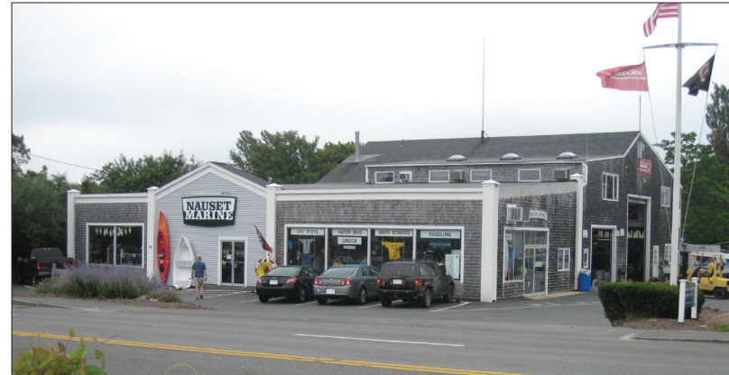
Figure B40: This building in Orleans uses traditional materials and incorporates traditionally scaled masses and roof forms close to the street to partially screen the larger building to the rear.
