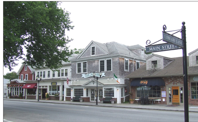
Figure A40: Relocating utility lines has reduced the visual clutter and improved the appearance of this portion of Falmouth Village (the top photo shows the area before the utility lines were relocated; the same area after utilities were relocated is shown above).
