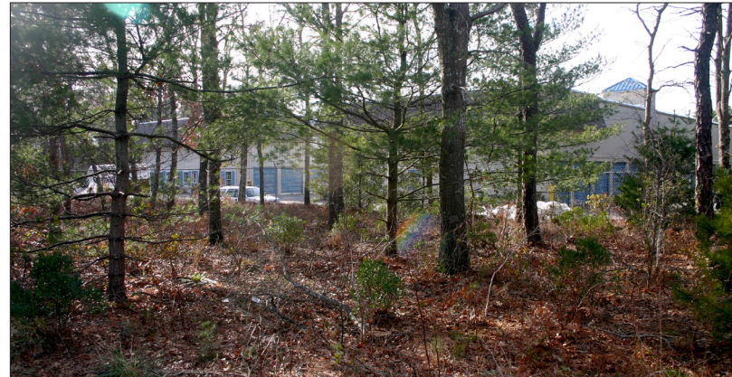
Figure A30: At this Mashpee storage facility, a wide natural buffer has been retained to reduce views into the project.
