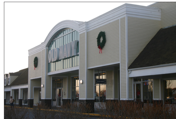
Figure B8: The entrance to this retail clothing store, located in a large commercial plaza in Hyannis, is defined by projecting the building mass forward, with the entrance element below the height of the main building.
