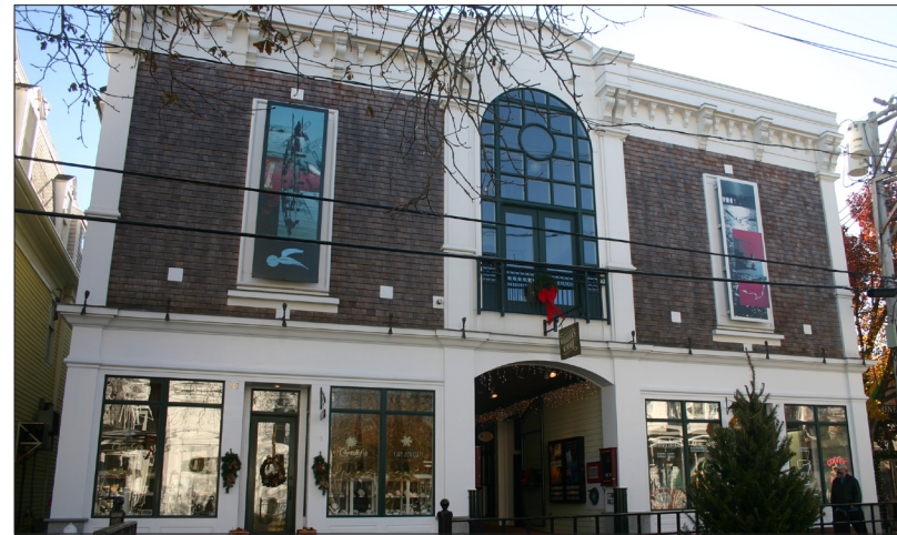
Figure A22: This reconstructed two-story commercial building in Provincetown incorporates large upper-level windows to allow light into the building.
