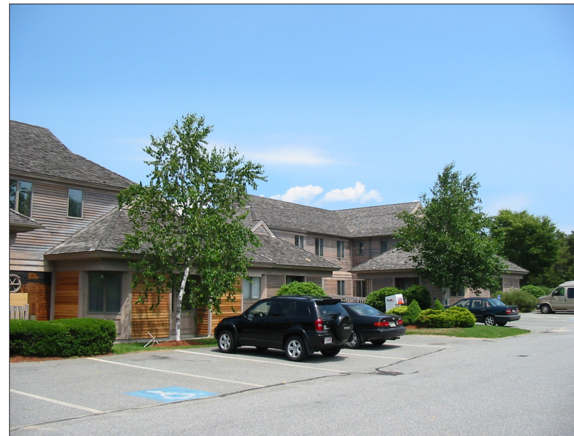
Figure B14: A combination of one- and two-story wall heights reduce the overall building volume in Mashpee.
