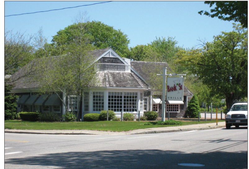
Figure A2: In this Harwichport example, the structure is oriented to the street establishing the street edge and "anchoring" the corner.
