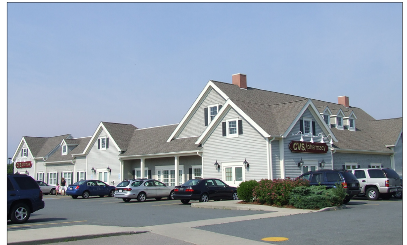
Figure B16: Roof peaks of various heights help to break down the building mass and effectively screen the flat roof in this Sandwich commercial building.
