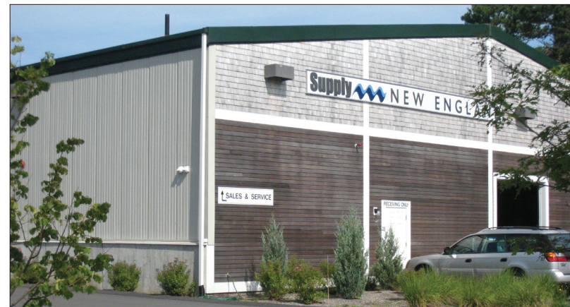
Figure B29: This building in Yarmouth uses a mix of traditional materials on the most visible facades and low-reflective siding in neutral tones on the remaining facades.
