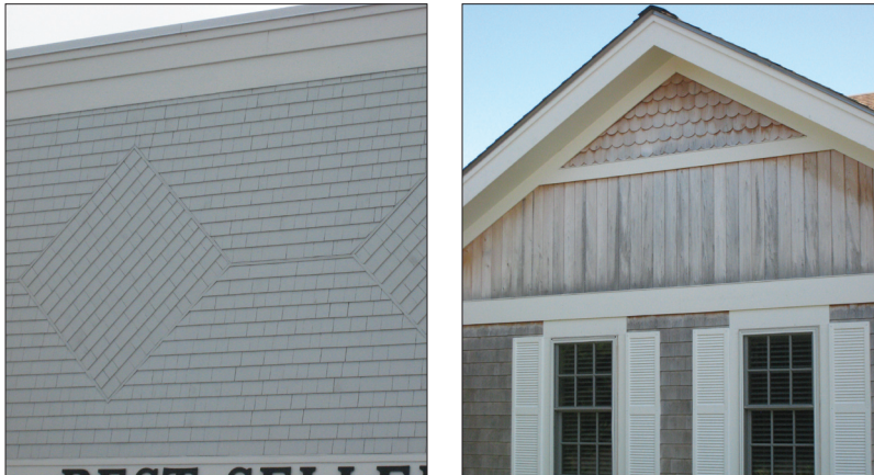
Figure B22: Simple changes in the pattern of the exterior materials and the use of bands of different materials can create interest in the facade, as shown in these Harwich examples.
