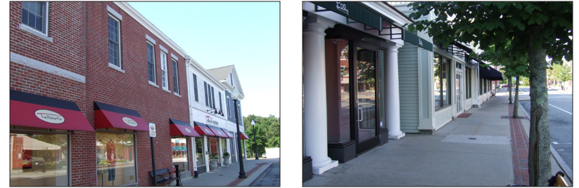
Figure B23: Different materials (clapboard and brick) and simple changes in the mortar colors (for brick cladding) in combination help break the plane of the facade into smaller components in Mashpee (left). Use of higher quality materials, display windows and varying architectural details creates a more-inviting pedestrian experience, also in Mashpee (right).
