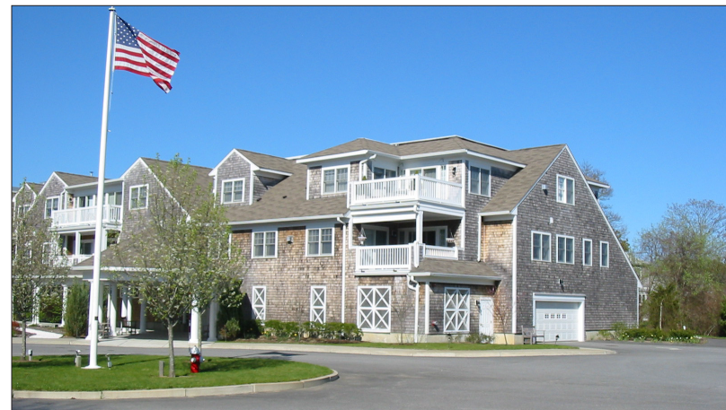
Figure A36: First-floor parking garage within residential multi-family building in Chatham.
