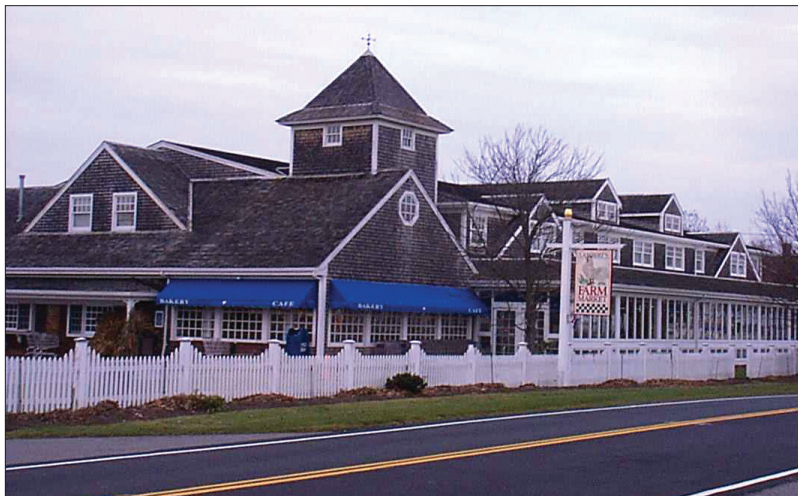
Figure B15: The varied rooflines of this Harwich building add visual interest.
