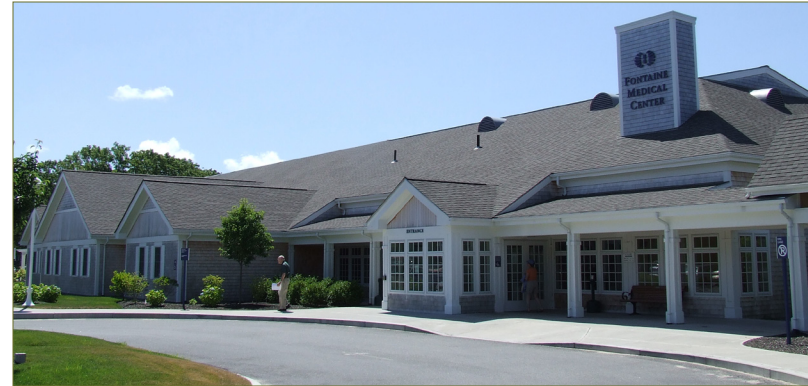
Figure B19: This medical facility in Harwich uses arcades, varied eave lines, and ridge heights to reduce the apparent mass of the building.
