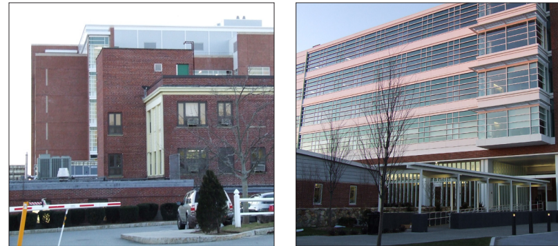
Figure B28: The addition to the Cape Cod Hospital (background center in the left photo) relates to the scale of the existing hospital buildings when viewed from the rear but presents a contemporary facade on the other side (right). The use of traditional materials and a complementary color palette tie the overall design together.
