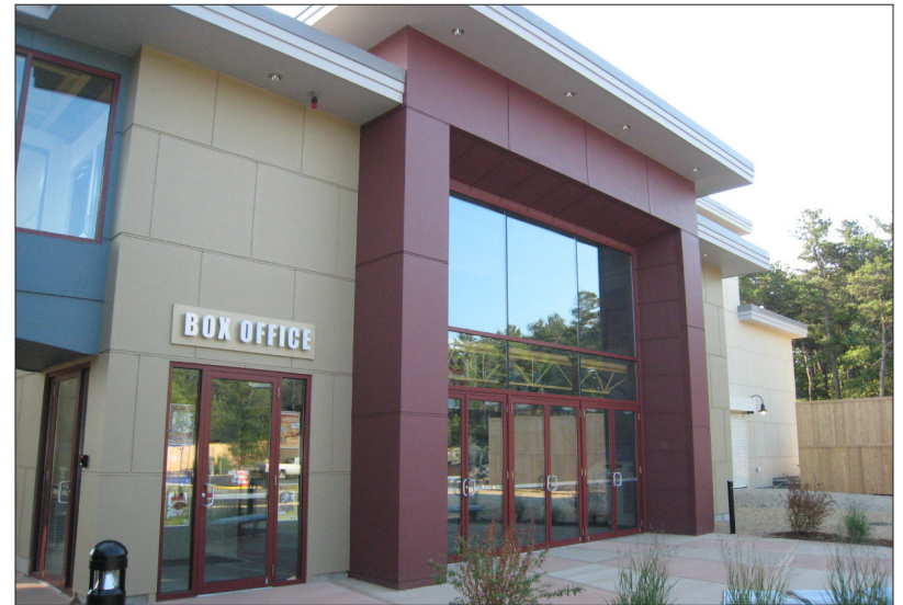
Figure B25: In areas not in village centers, the use of non-traditional materials may be appropriate. At the Wellfleet Harbor Actors Theater in Wellfleet, the use of non-traditional materials in combination with changes in color and mass are consistent with the more-contemporary style of the building.
